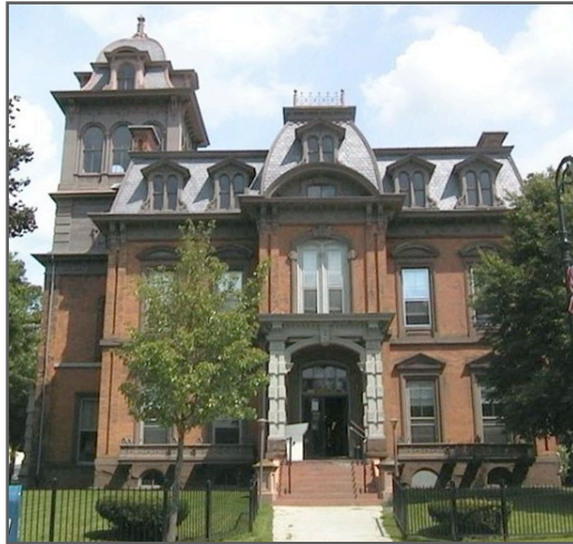
The North Adams Public Library is a model of green building design and the public face of Take Charge.
