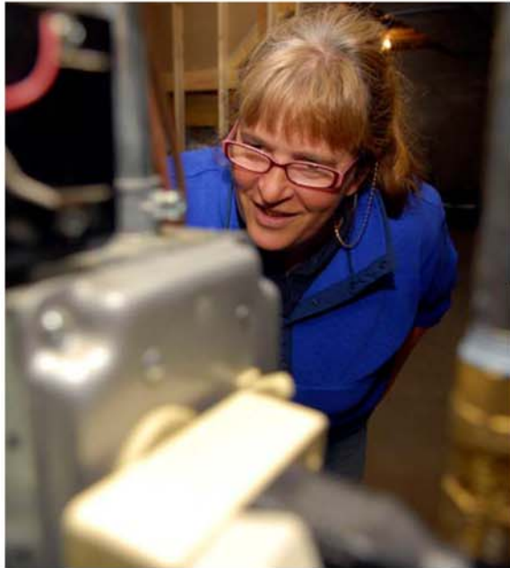
A green home specialist performs combustion safety testing
