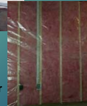
Friction Fit Fiberglass With Vapor Barrier
