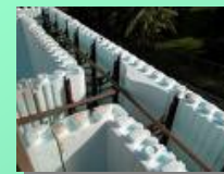
ICF's Insulated Concrete Forms
