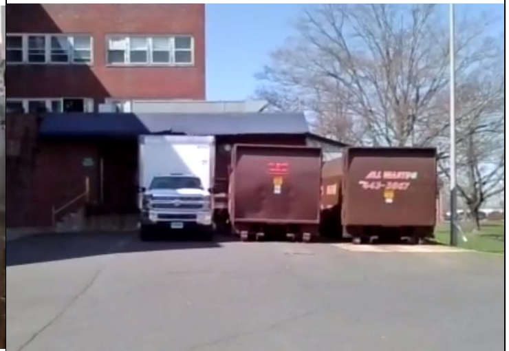
Loading dock with trash and recycling compactor.
